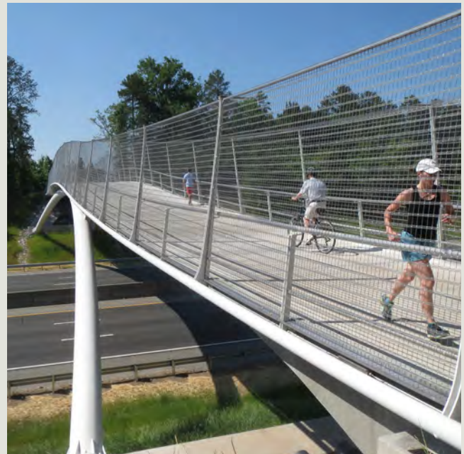
Grade separated crossing at I-40 on the American Tobacco Trail in Durham
